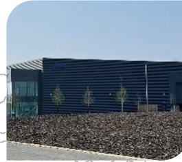
Harlow, UK customer support & design center
